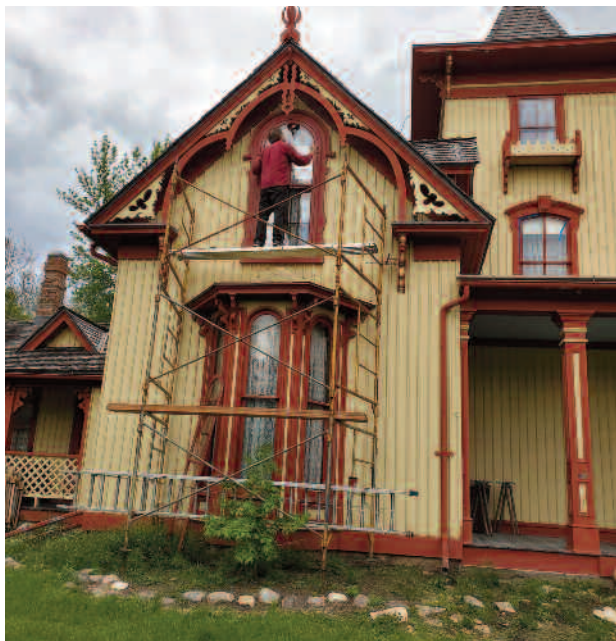
Storm windows are being repaired and re-installed by NCHS member and local craftsman Eric Hendrickson.
