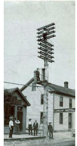
This photo shows two St. Peter linemen working with the electrical connections on a power pole in front of the Strehlow Hotel at 216 and 218 Nassau Street in St. Peter. The neighboring Walter Cigar Factory was at 212 Nassau Street and was owned by John Walter, Jr.
