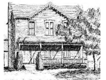
Old Anderson House Minnesota & Broadway circa 1870s moved from St. Peter in 2009
